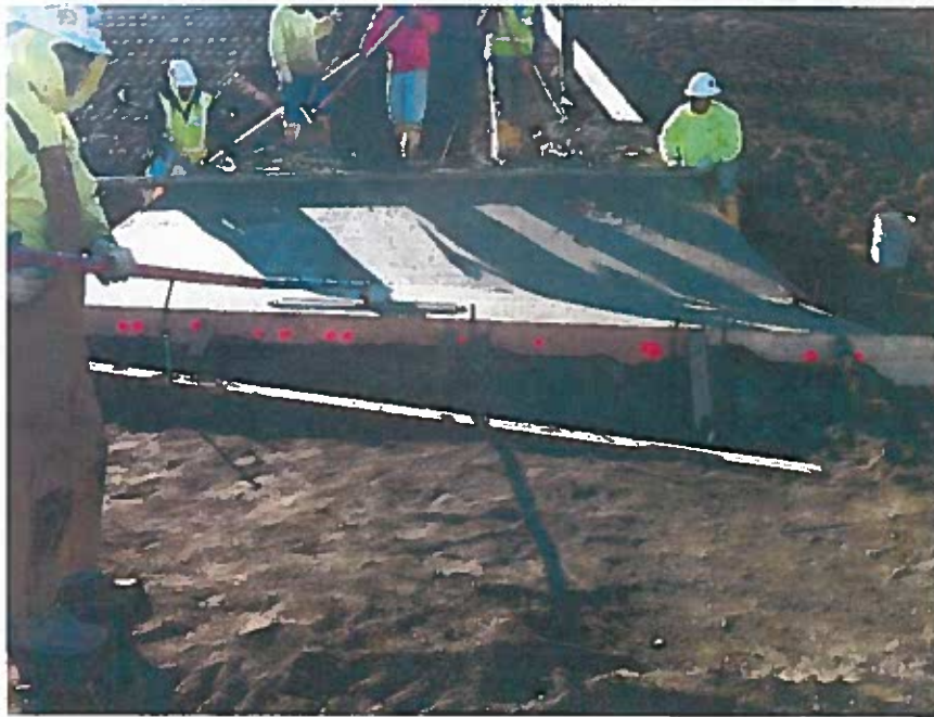
View of the construction of the concrete apron.
