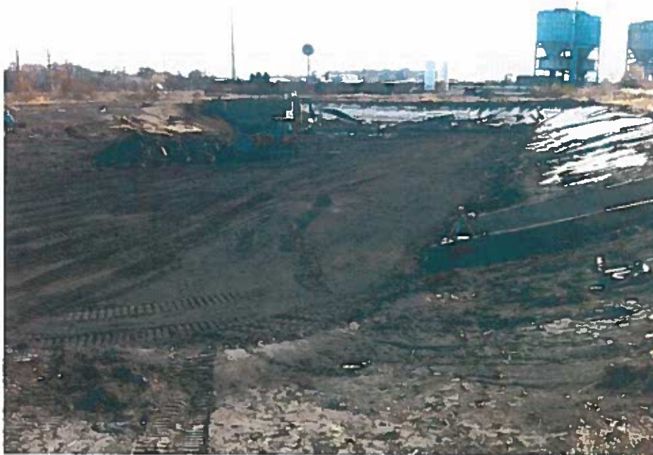
View of pozopac load out and subgrade preparation.
