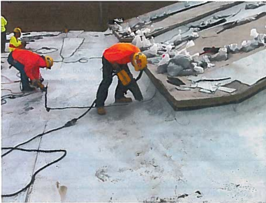
View of extrusion seaming around aprons.
