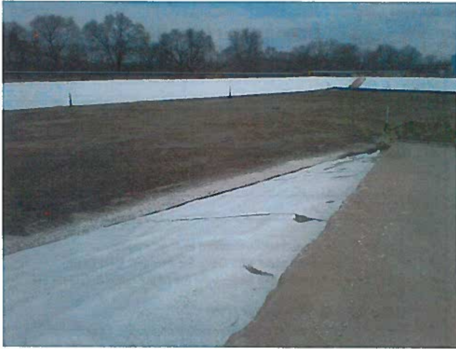
View Looking Northwest Along Ramp.
