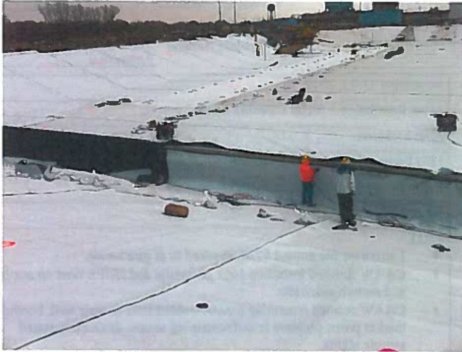
View of liner being attached to weir wall HDPE weld strip.
