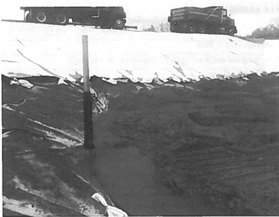
View of soft spots and ponding in the northern portion of the basin.
