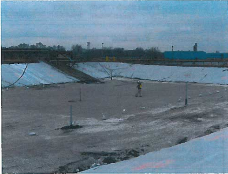
View of the bypass basin during the leak location survey.
