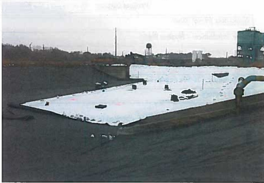
View of 16 oz geotextile in place and HDPE liner being placed.
