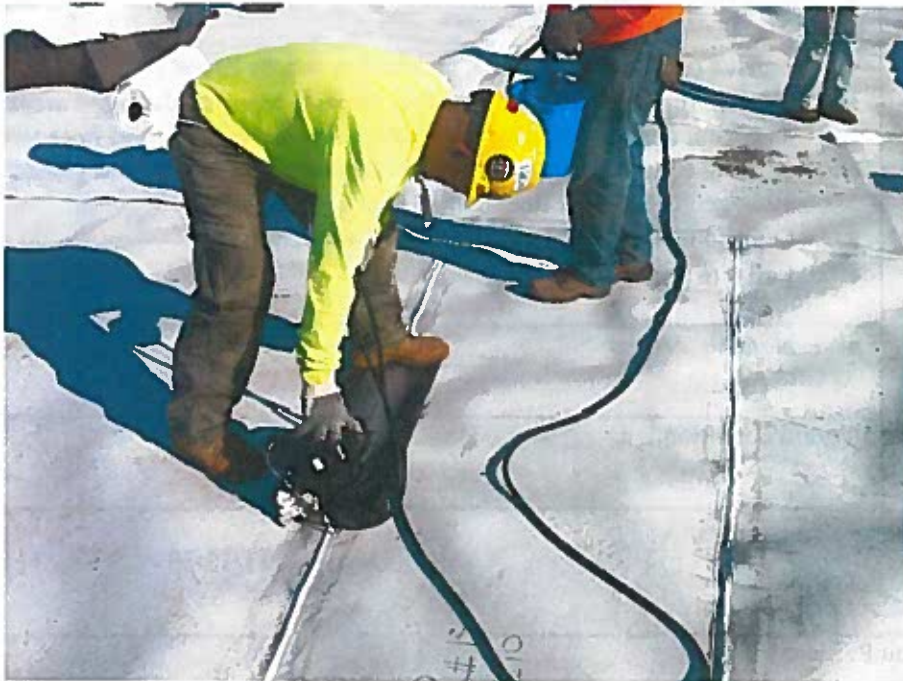
View of extrusion seaming vacuum testing.
