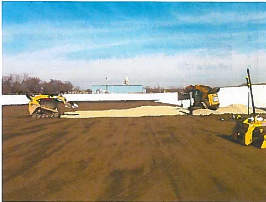
View of finished cushion layer and beginning of warning layer.
