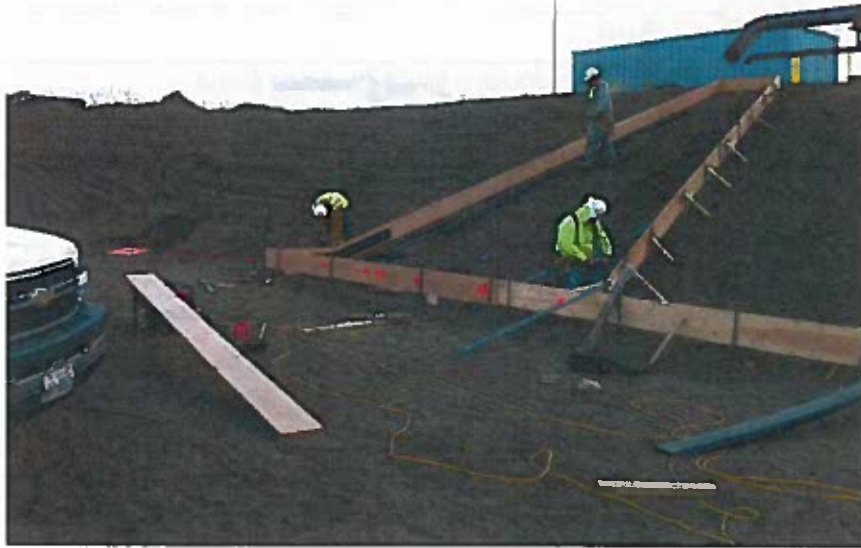
View of the concrete apron forms. Note HDPE weld strip.
