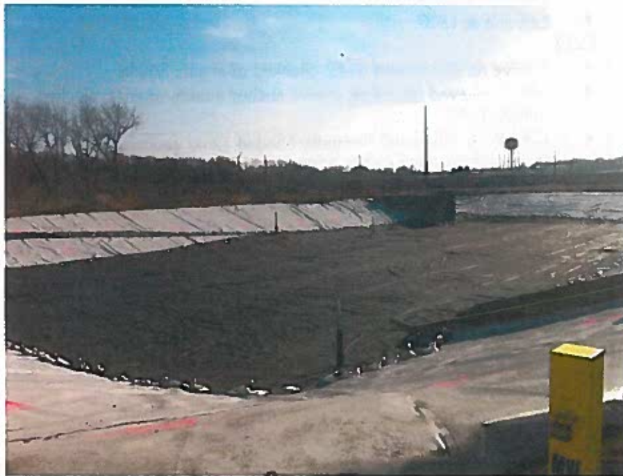
View of finished liner with finished 12 oz geotextile .
