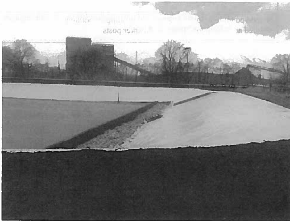
View of finished rip rap north of weir wall.
