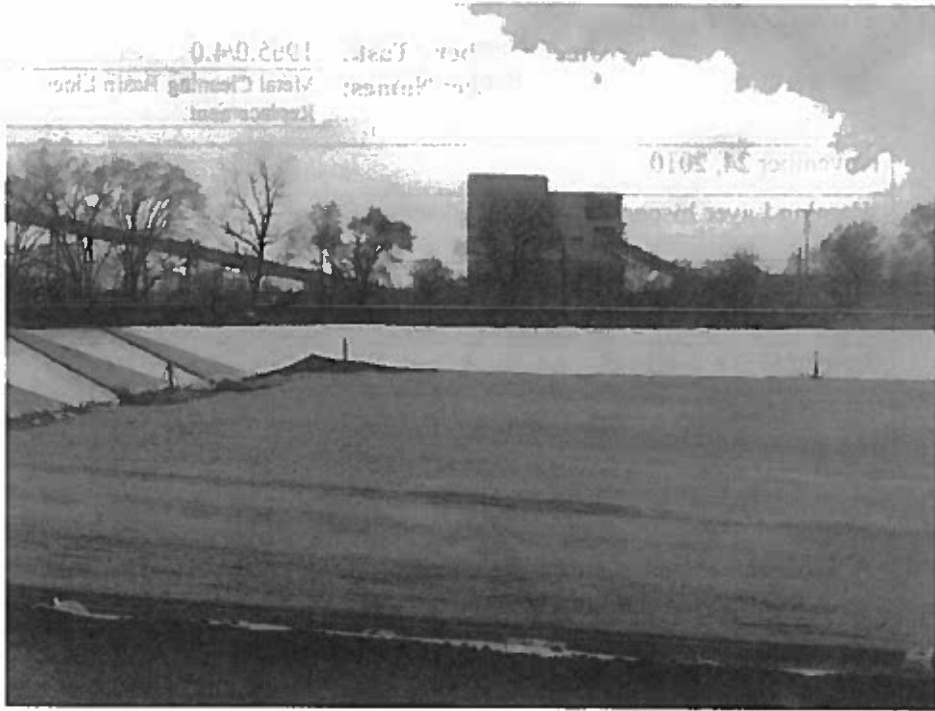
View of warning layer in the southern end of basin where additional cleanup and finishing is required.
