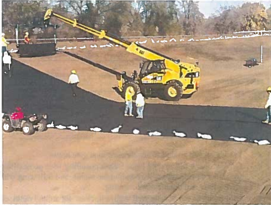
View of 16 oz geotextile being placed on the western slope and thermally bonded at the seams.
