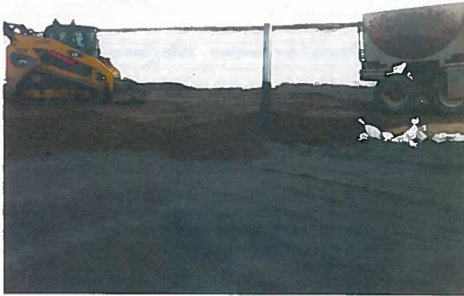
View of liner placement of cushion layer sand.
