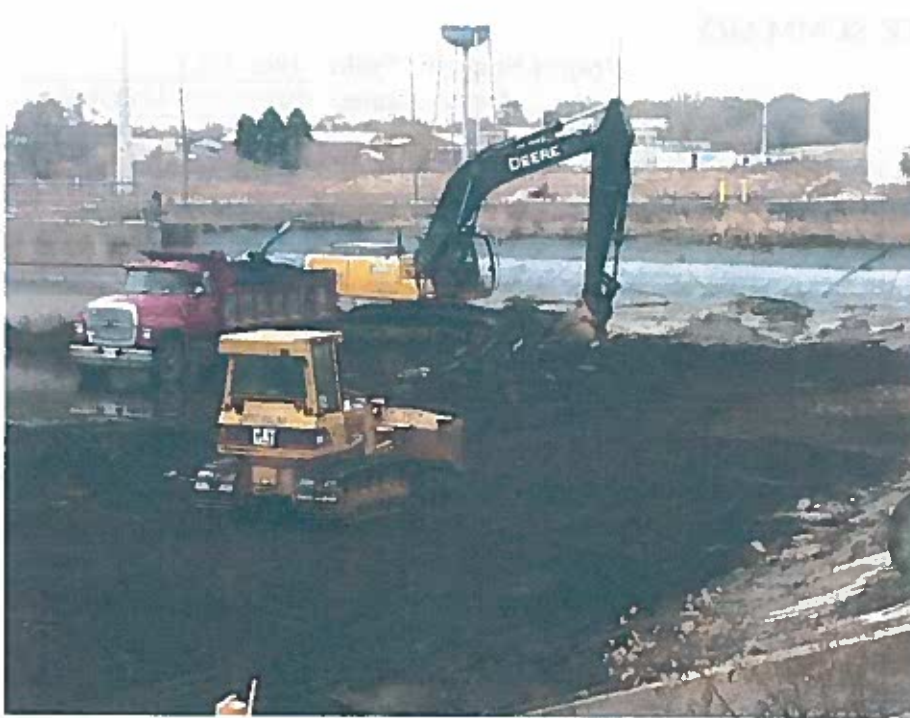
View of pozopac removal and subgrade preparation.
