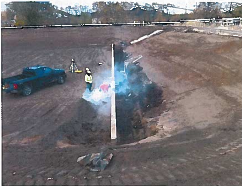
View of excavated weir wall during steel gate removal.
